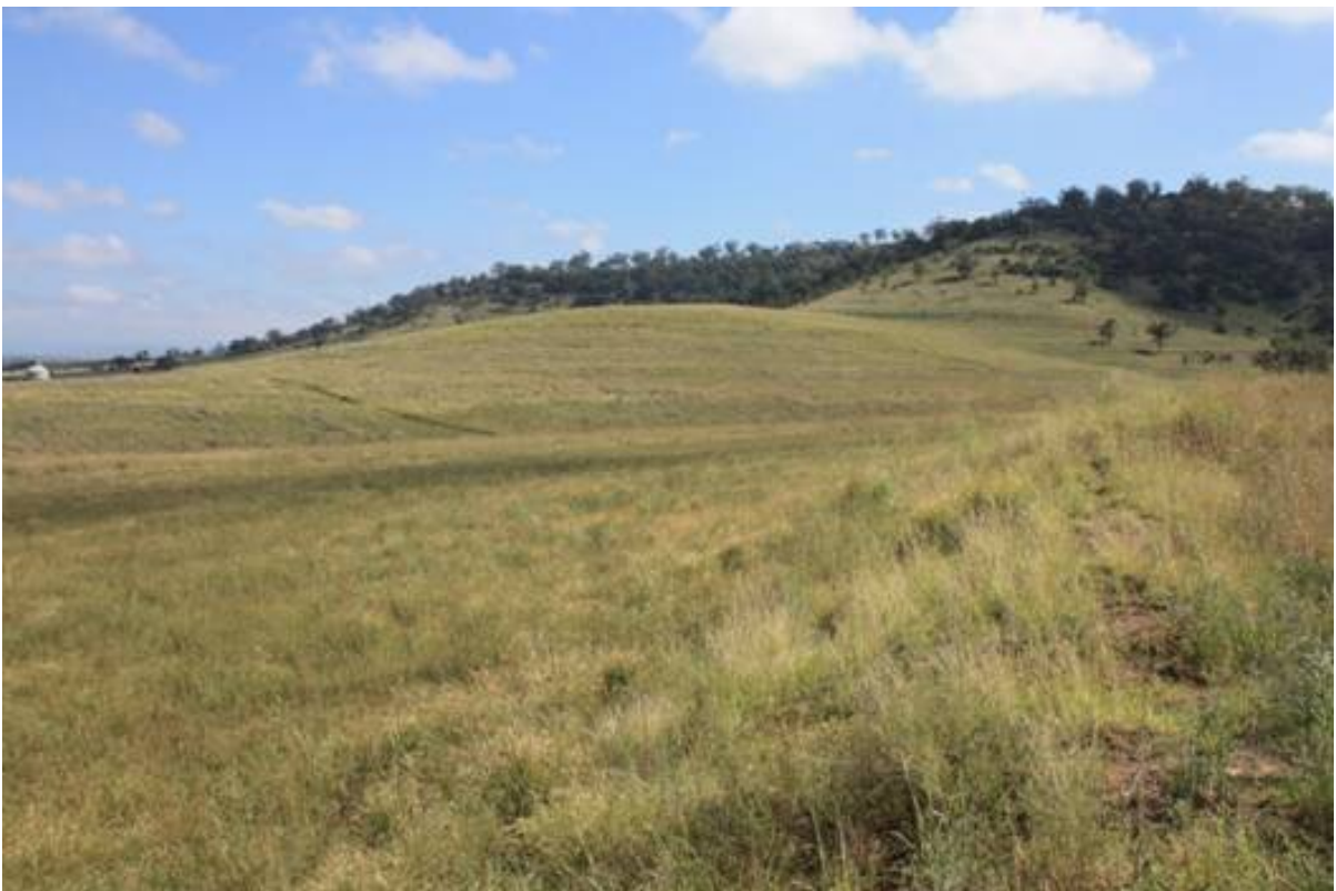
Plate 2 – REA rehabilitation 2010 - Western slope looking uphill to the northeast.
